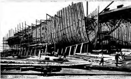
Two of the vessels building at the Peninsula plant in frame and scribing frame sections on large timber slabs.
